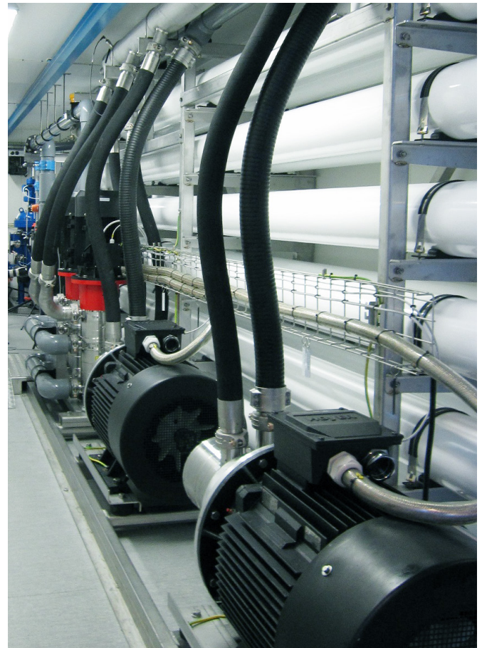
Containerized unit built with 2 APP 30 pumps and 2 iSave 40. Photo: Enwa Water Treatment.
