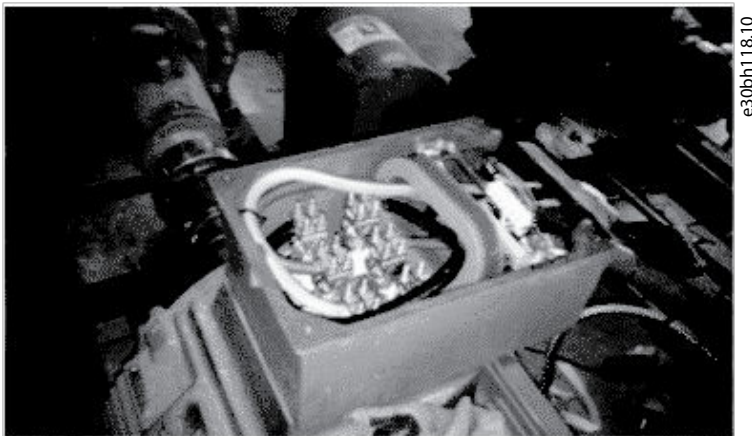
Illustration 20: Mounting of CM Cores Inside the Motor Terminal Box
