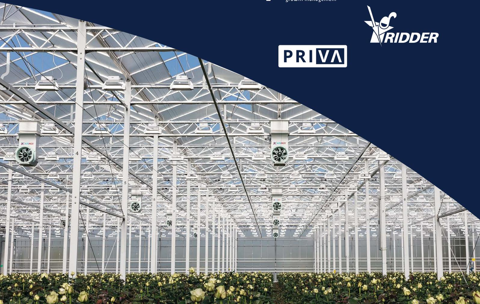
The Airmix allows active ventilation with a closed screen by blowing air from above the screen into the greenhouse below the screen. The purpose of this active ventilation is different in each greenhouse. In some situations the greenhouse temperature needs to be reduced, while in others the aim is to remove moisture so that evaporation is maintained. Both of these are possible because the temperature and absolute humidity of the air above the screen are generally lower than below the screen.
